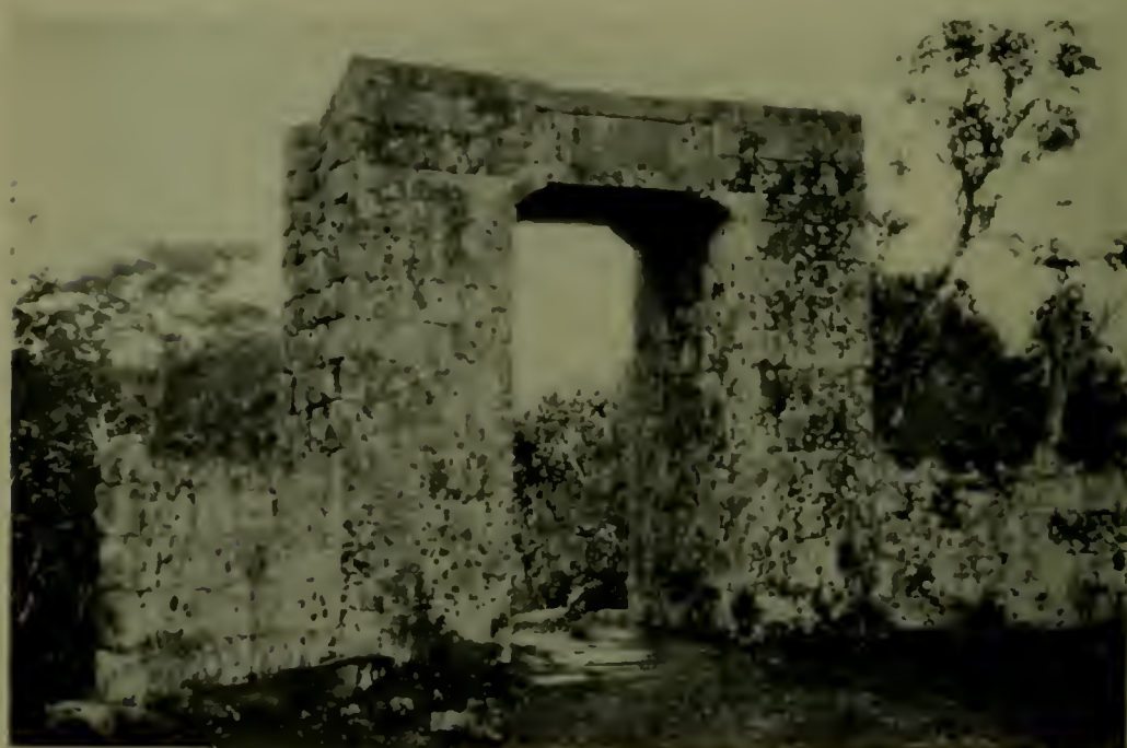
In the region of the coastal Loi of Hainan all villages and many estates have great gateways made of the lava-stone with which the district is overrun
